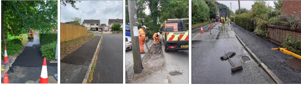
Footway renewal programme resumed in the summer
