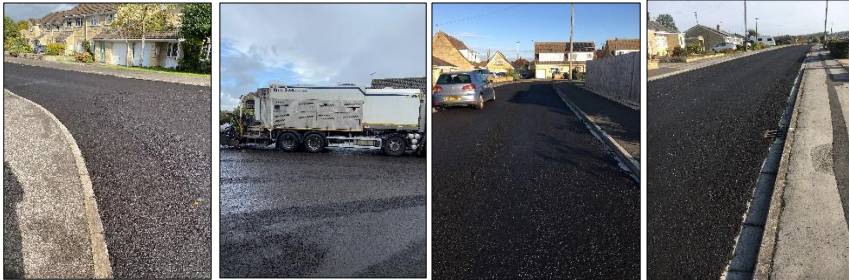
Microasphalt surfacing was carried out by new contractor Kiely Brothers
