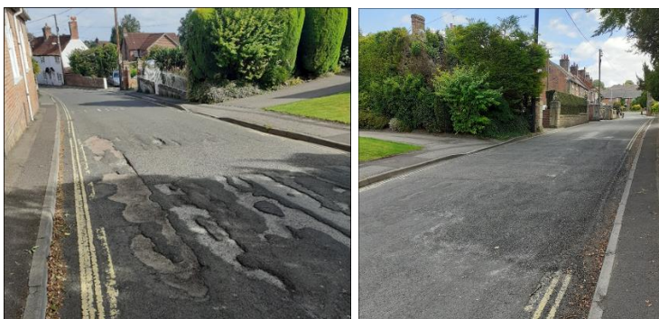
Before and after Jet Patcher repairs in Westbury.
